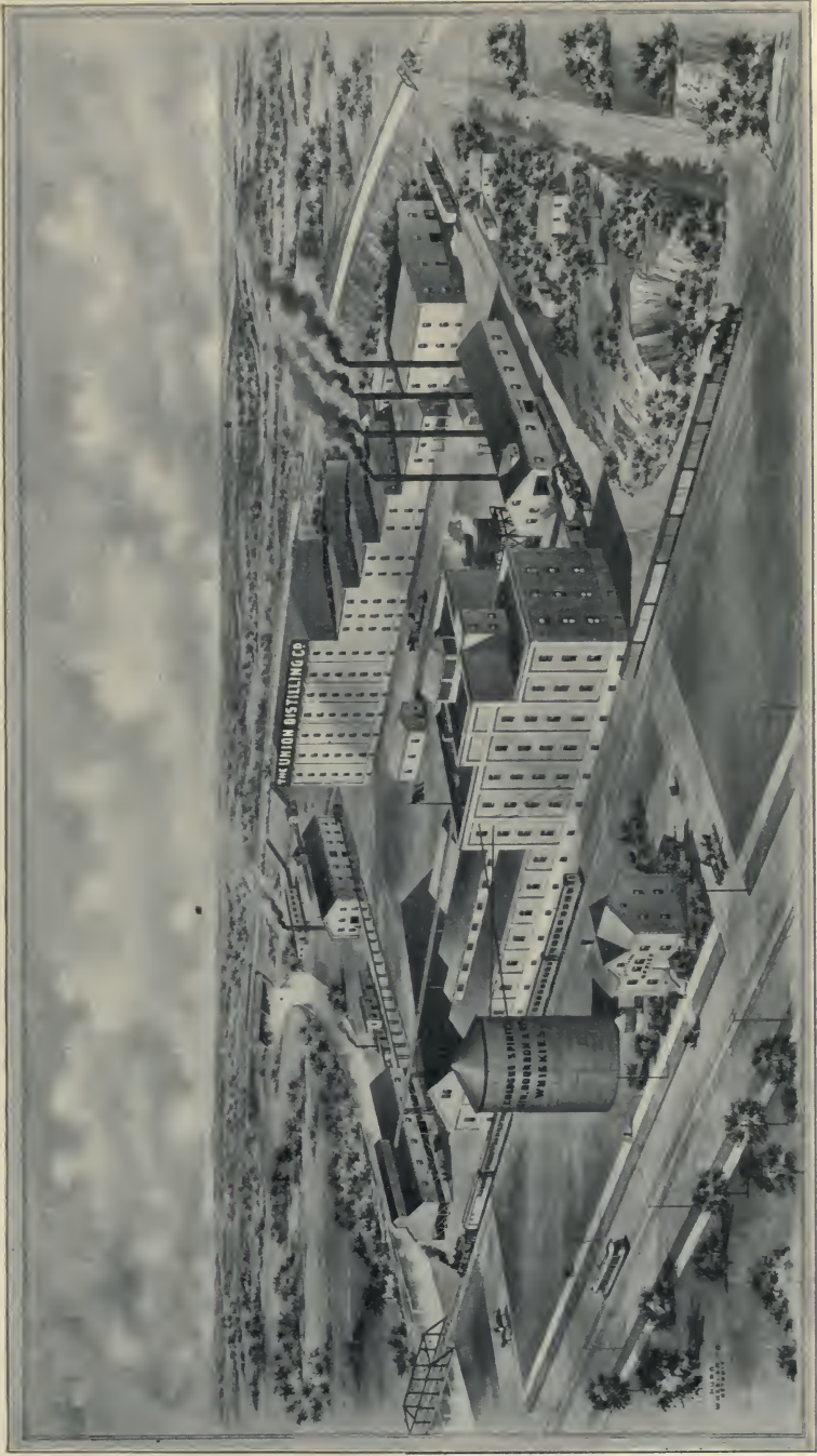
FIG. 73.—A Model Distillery (capacity 5400 bushels per day). Owned by The Union Distilling Company, Cincinnati, Ohio, Manufacturers of Denatured Alcohol, Grain Spirits, and Grain Alcohol.
