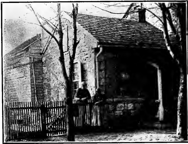
OLD LANDMARK, FORMERLY THE HENRY PETERSON HOME, WEST WHITEOAK ST.
