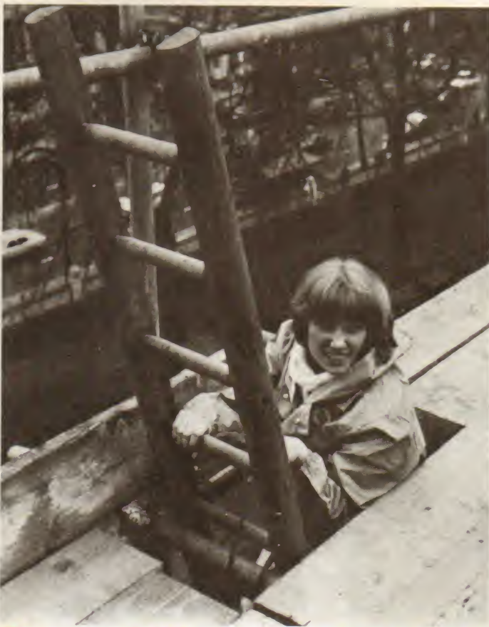
The museum's 200-metre frontage was covered with a network of scaffolding and interconnecting ladders.
