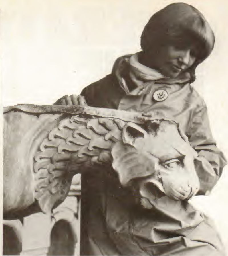
Gargoyles like these aren't just for decoration. Inside they contain drainage troughs and pipes to stop the rain damaging the walls.
