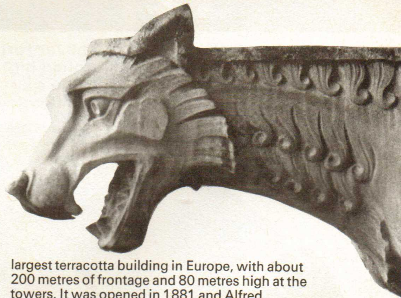
Gargoyles like these aren't just for decoration. Inside they contain drainage troughs and pipes to stop the rain damaging the walls.
